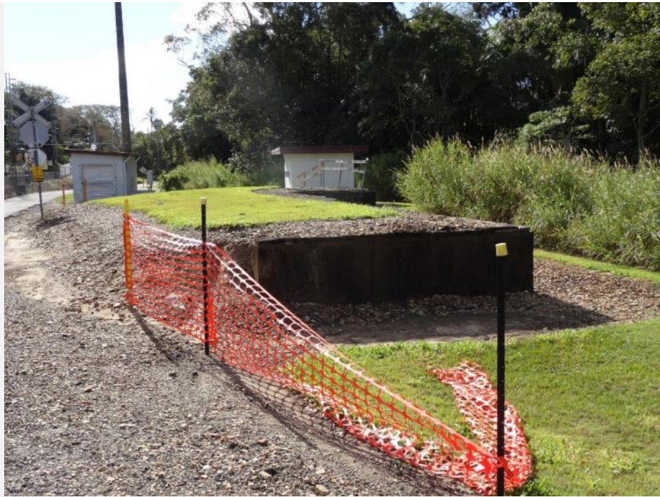
Plate 41. Palmwoods Station earth and concrete loading banks north of the station and siding.
