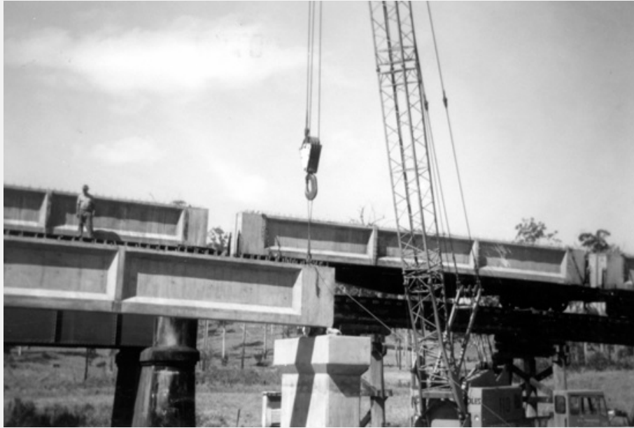
Plate 31. Construction of new bridge in 1965; noted concrete piers and timber piers of earlier bridge behind (Source: JOL collections).
